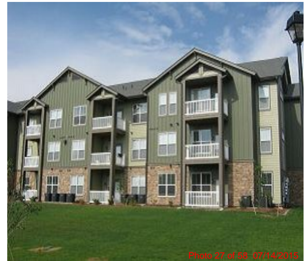
Building 11 from the patio
