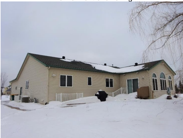
View of rear of dwelling
